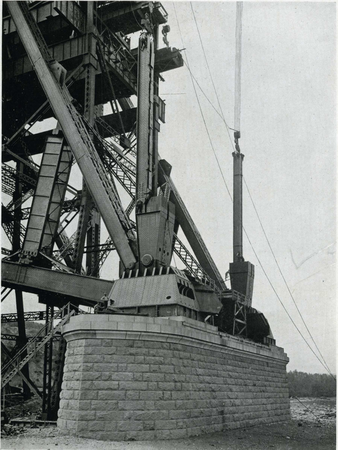
23—Starting the erection of the anchor arm web system
